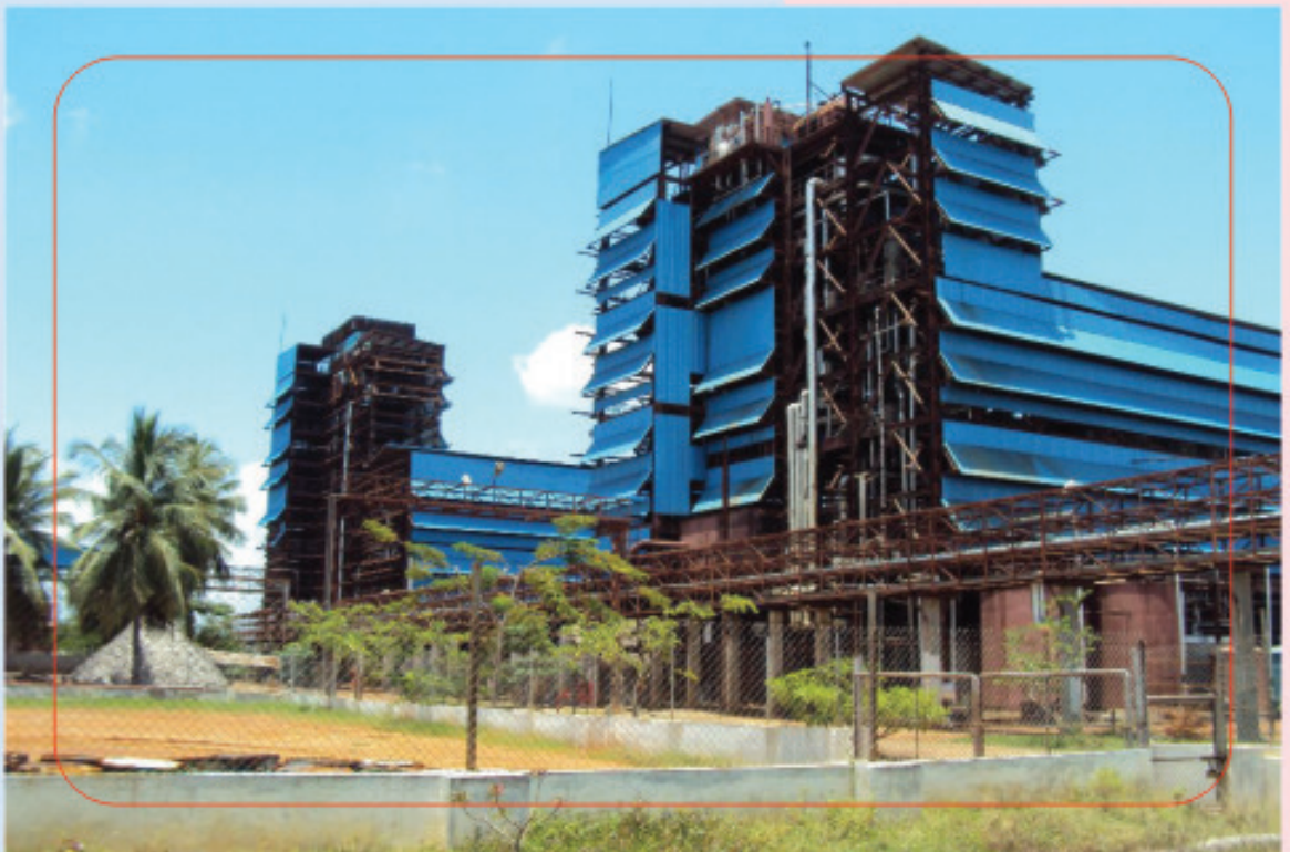
SBT Biodiesel Plant - Visakhapatnam
