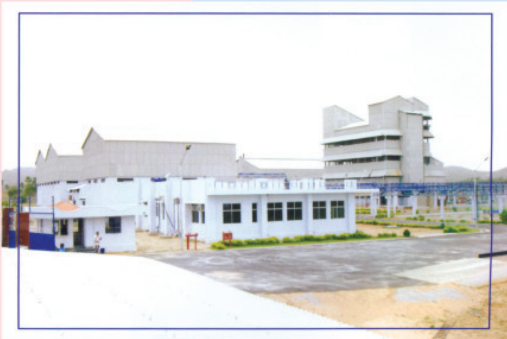
SBT Biodiesel Plant - Samsthan Narayanpur (Village & Mandal), Nalgonda Dist.,
