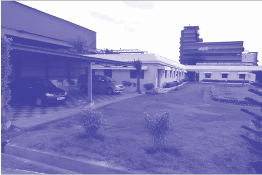
SBT Biodiesel Plant – Visakhapatnam
