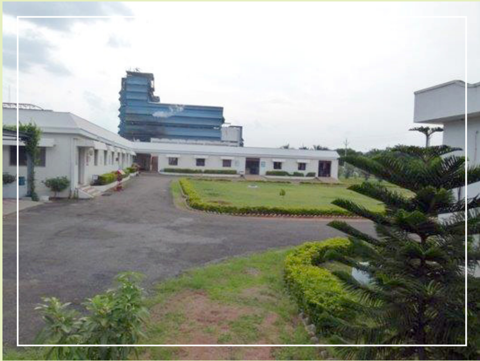
SBT Biodiesel Plant - Visakhapatnam
