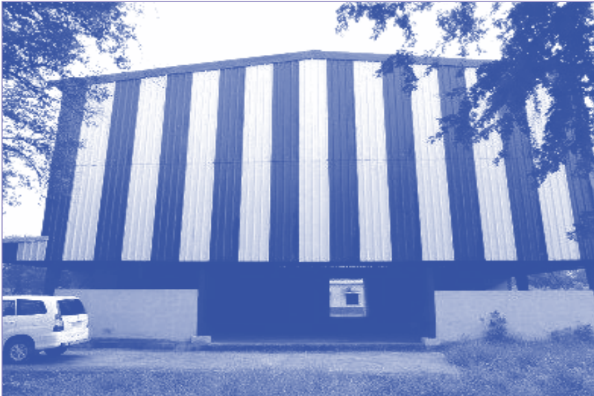
IROAF (Indian Railways Organisation for Alternative fuels) 30 TPD Biodiesel Plant at Raipur, Chattisgarh Under implementation by SBTL
